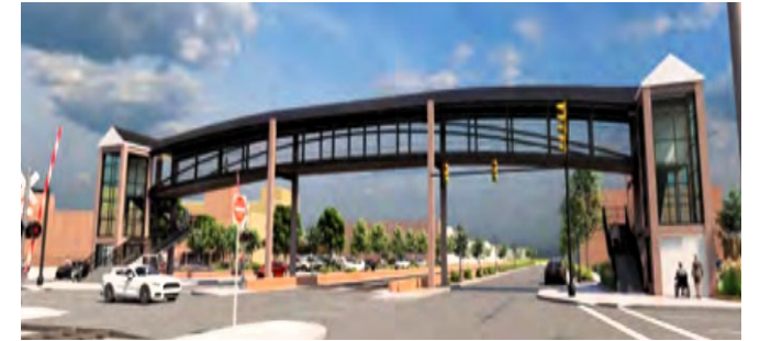
Rocky Mount – Planned Pedestrian Bridge over a CSX RR. Rocky Mount Telegram
